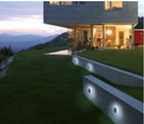
PATH INDICATORS ON DRIVEWAY
